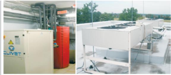
**Figure 3.** Chiller, coolant pipes, coolant vessel and remote air cooled condensers
