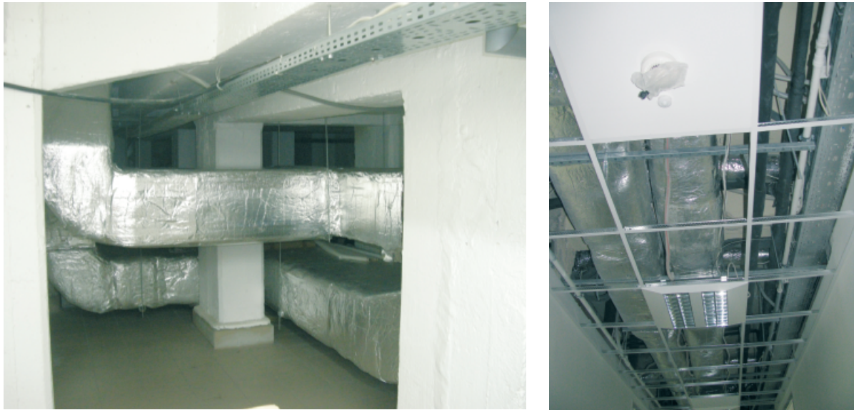
Figure 1. Insulation of ventilation ducts: in the engine room (left), in the suspended ceiling (right)
