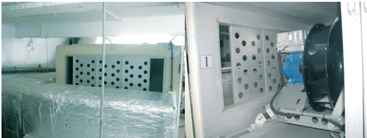
Figure 2. The pressure adjusting plates on exhaust opening of air handling units: view from the outside (left), view from the inside (right)
