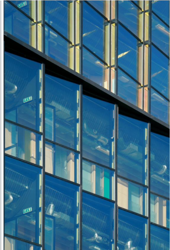
Figure 7. Music Conservatorium of Amsterdam (arch. van Dongen – Koschuch, 2005). Originally published in [2]. Photo by author
