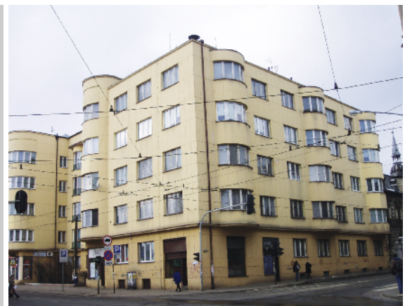
Figure 7. Corner tenement-house – 55 Gdańska / 25 Zielona Street, intersection side view (photo by the author, 2006)
